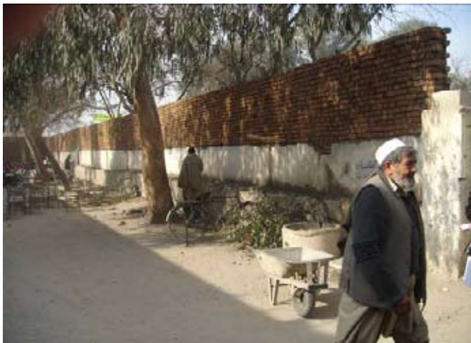
The school surrounding wall is about (50metere) long and (1.5metere) high built on the old one (first construction)
