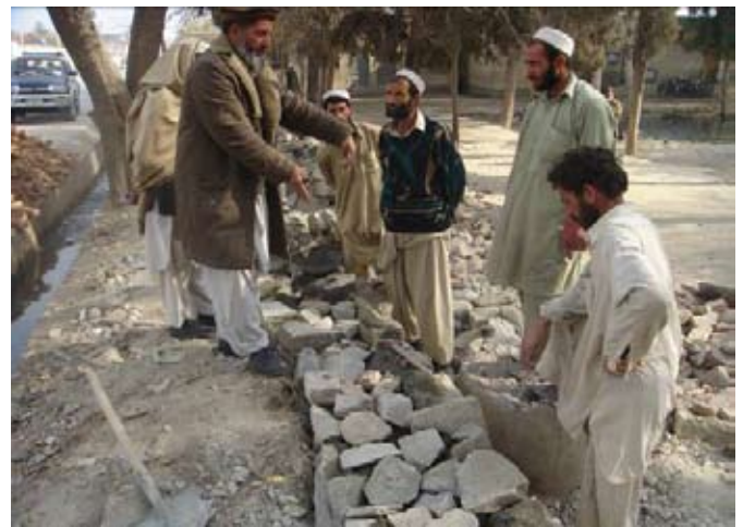
PTSA members instructing the workers for the rebuilding of school surrounding wall, (2,5metere) high (second construction)
